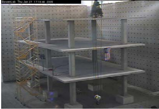
Fig. 2. An instrumented test infrastructure at the Bowen Labs (three story 30' \times 50' structure) with extensive actuation and response testing capability
